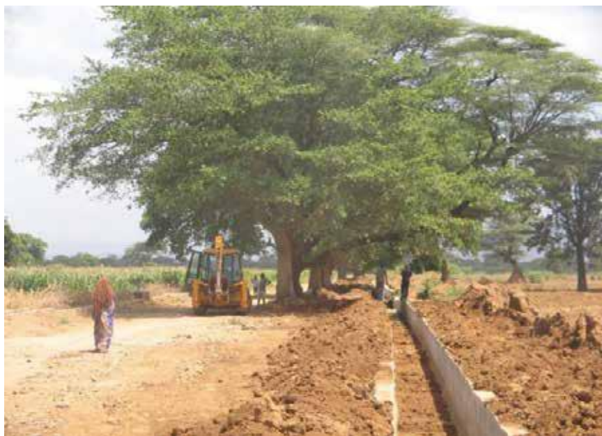
Plate 5: Construction of roads and laying of water pipes in an irrigation site
