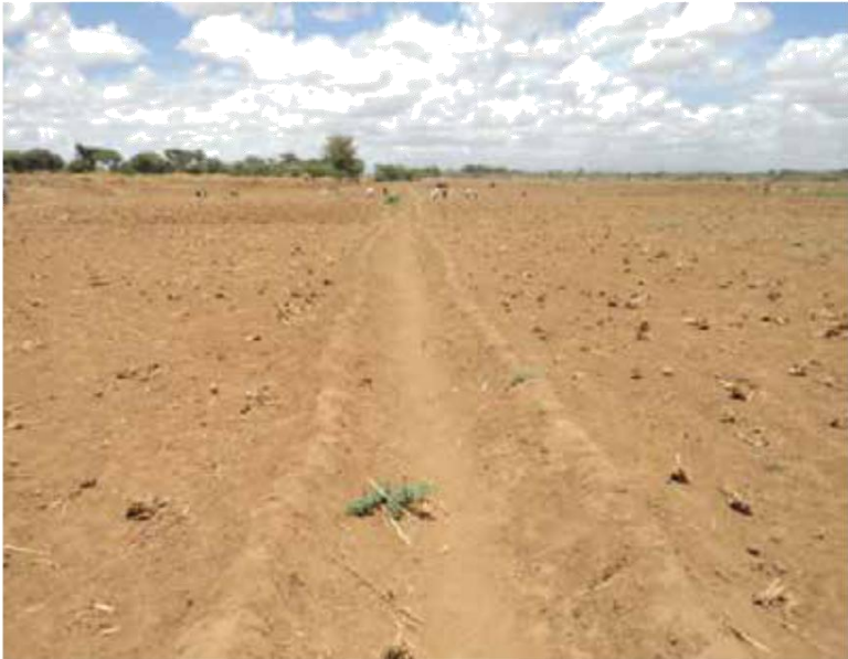
Plates 2 and 3: Vegetation clearing and land leveling to create conducive irrigation environment at Katilu and Nanyee irrigation schemes in Turkana County (Photo: Jesse Owino)
